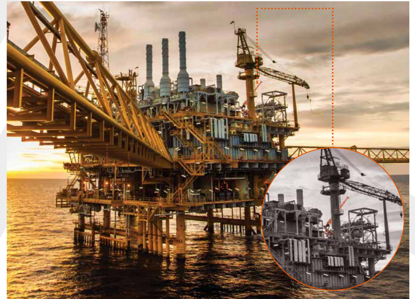
SPX312, working on an oil plant
